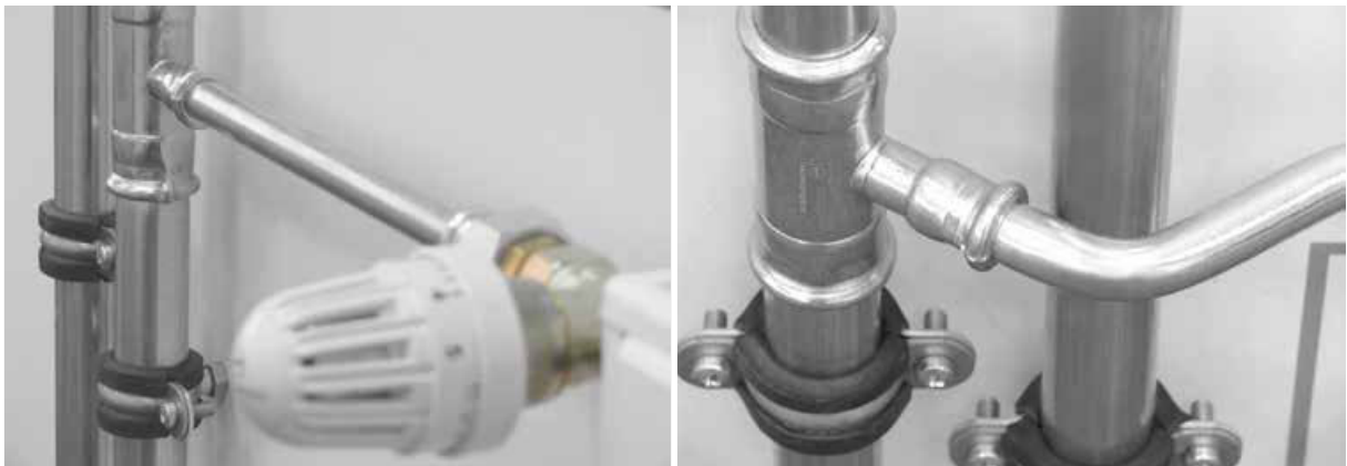
Radiator connection (connection pipe and return pipe) in the KAN-therm Steel system
