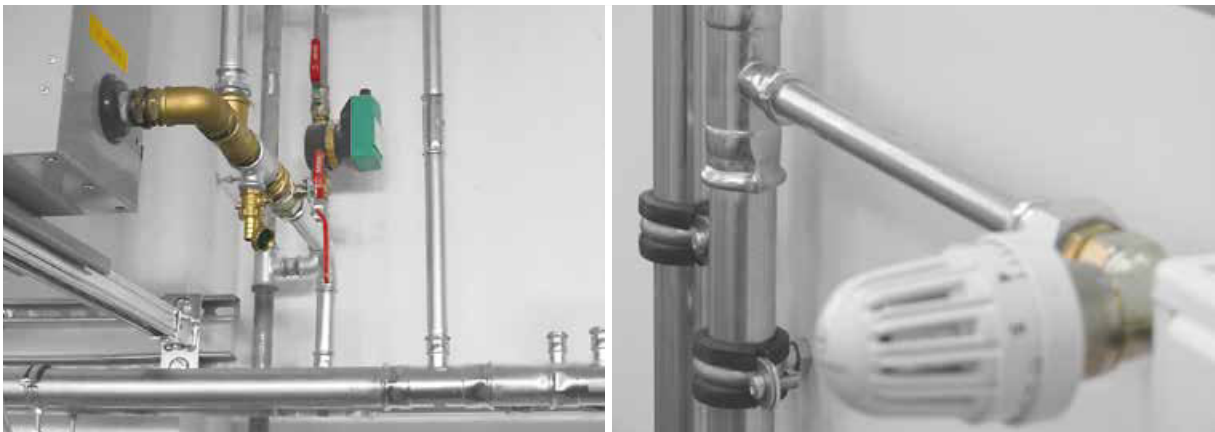
Examples of KAN-therm Steel installations
