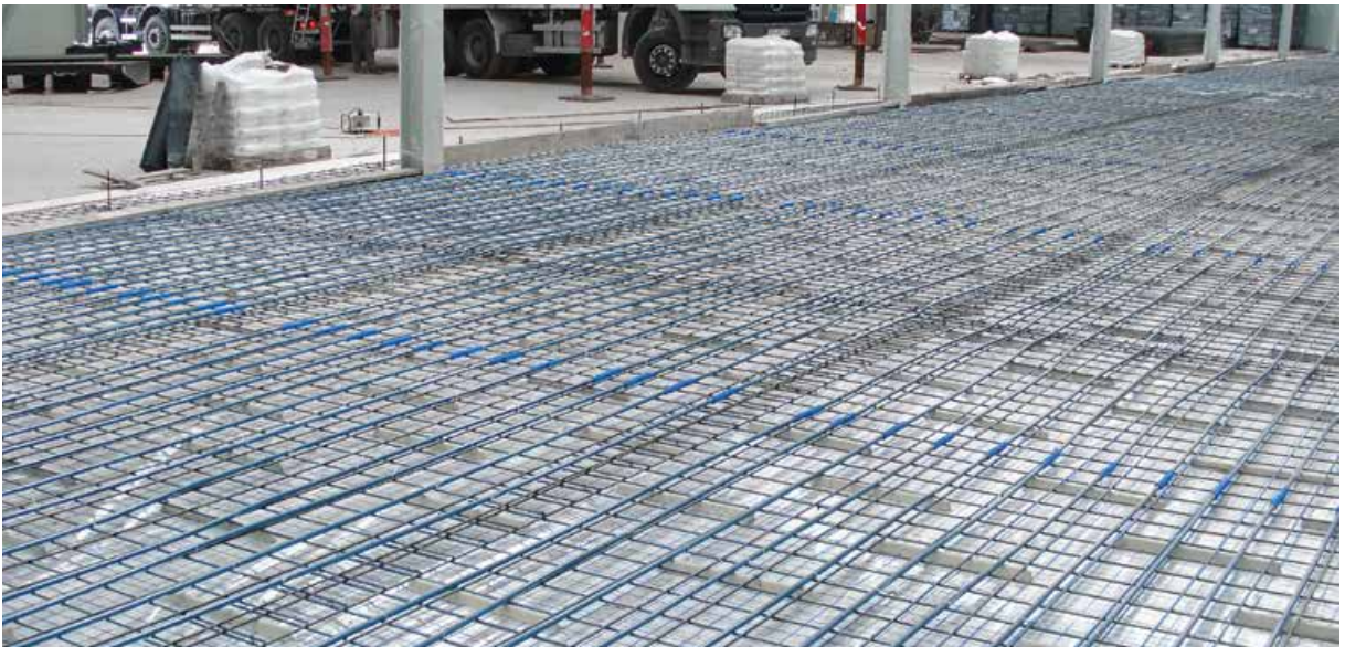
Fig. 4. Floor heating installation in industrial facility, employing bluePERT pipes and KAN-therm NET system.
