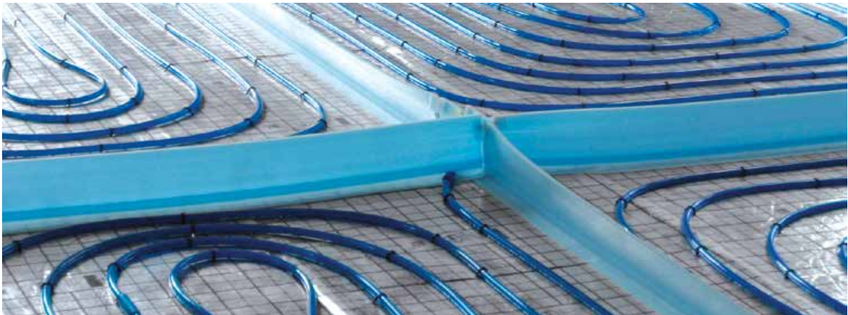
Fig. 14. Distribution of heating fields with dilatation gaps
