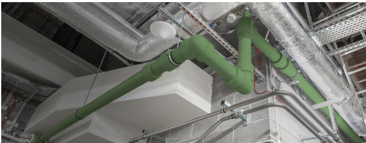
KAN-therm PP Green installation
