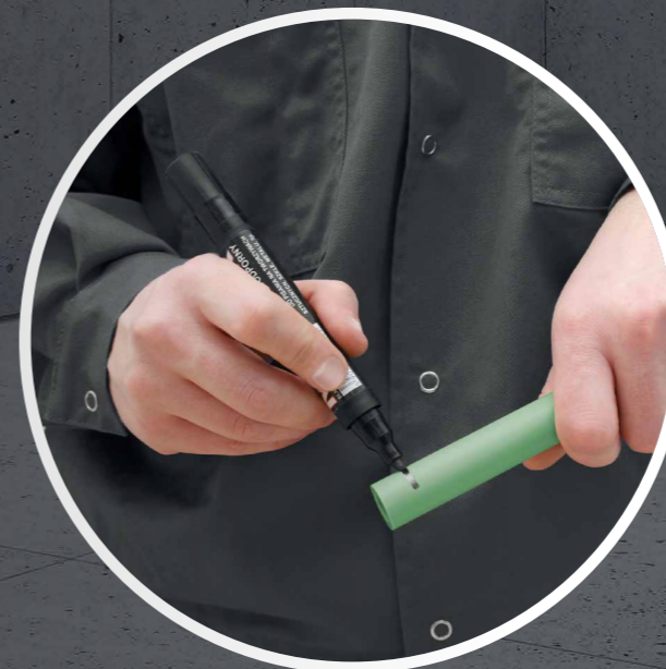
03 Marking the welding depth.
